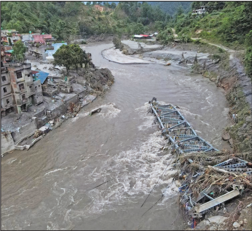
A drone view shows a broken bridge and damaged houses after the flash floods and mudslide, at Devighat, Nuwakot district, Nepal, on Aug. 28. (OSV News photo/Francis Mascarenhas, Reuters)
